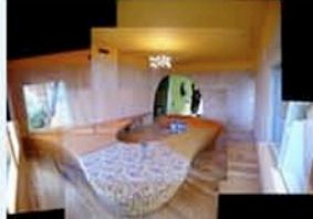
Bernardi Residence / Silverlake Hills, Los Angeles / under construction, to be completed summer 2007 / view of gathering room Photo: Fritz Haeg
