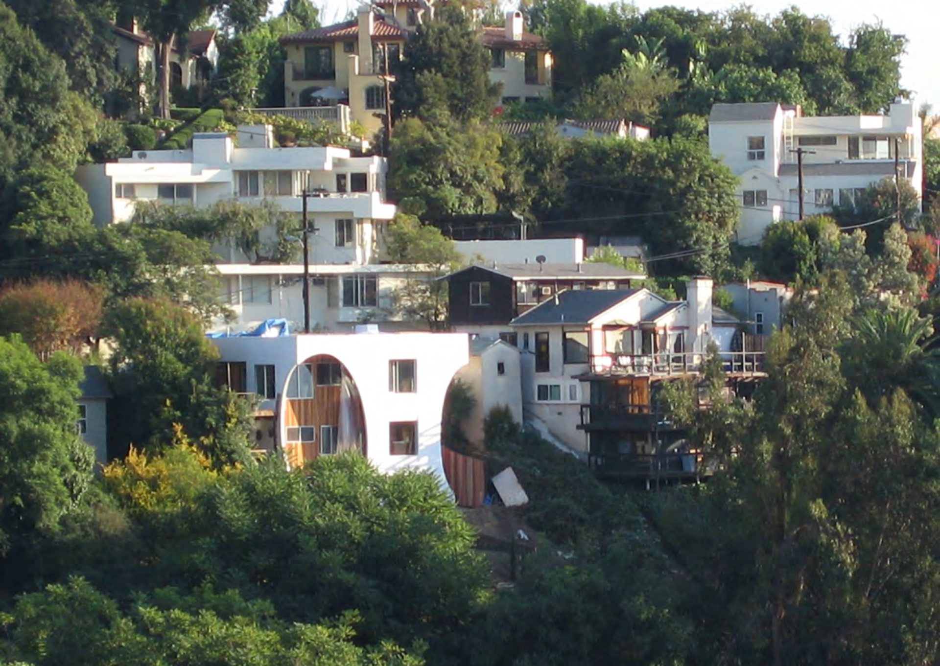
under construction as viewed from across the valley
